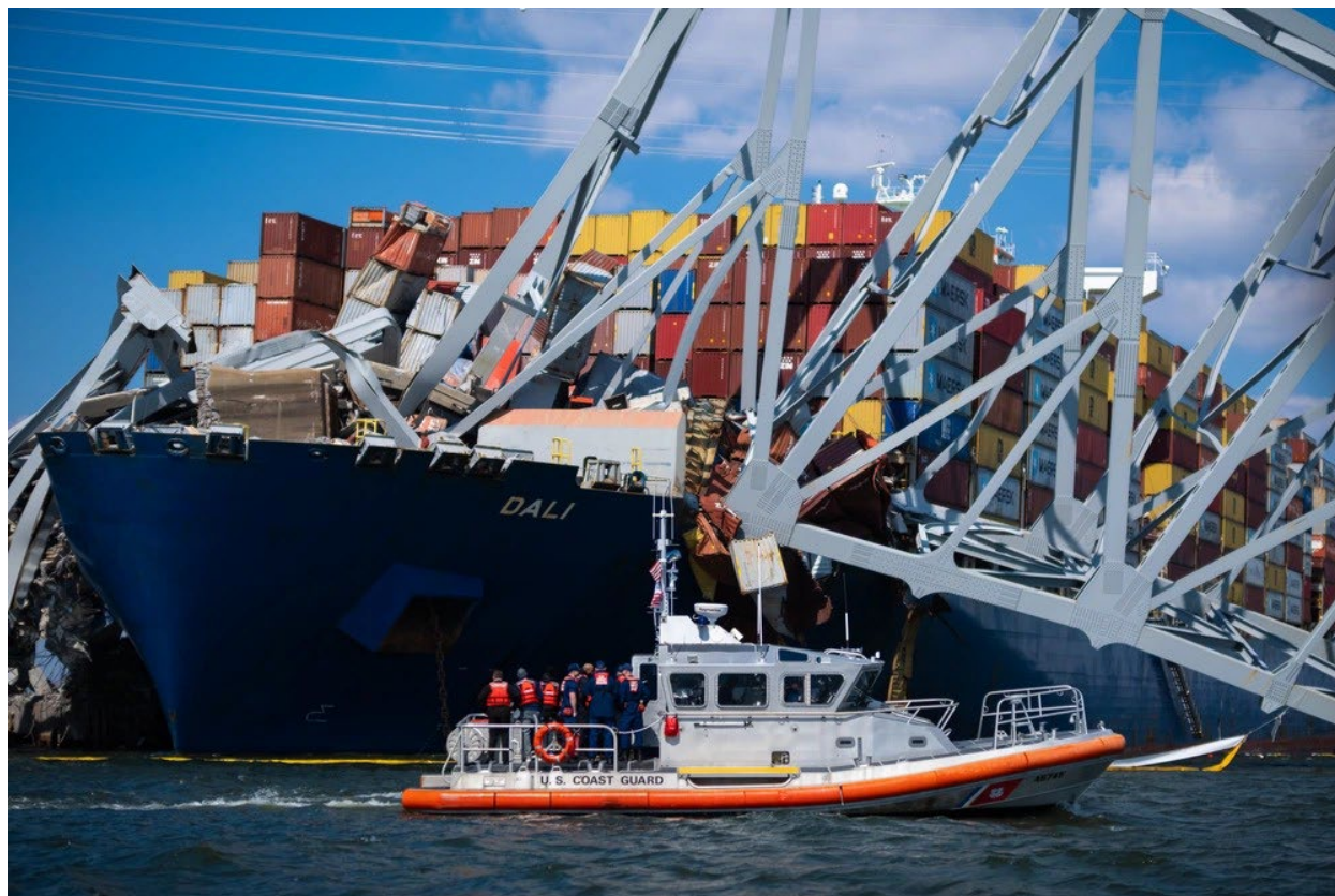
Figure 24: The Commandant of the Coast Guard, Governor of Maryland, and Mayor of Baltimore, transit by Coast Guard boat to assess the Francis Scott Key Bridge collapse in Baltimore, Maryland, March 29, 2024.
